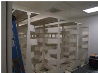
INSTALLATION OF ROLLING COMPACT STORAGE FOR ARCHIVES
