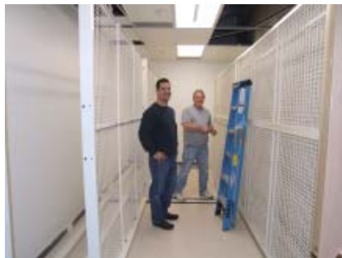
WORKERS INSTALLING FRAMED ARTIFACT STORAGE RACKS
